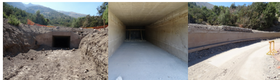
Andina Division: building new tailings transport system. Scheduled for winter 2017.
