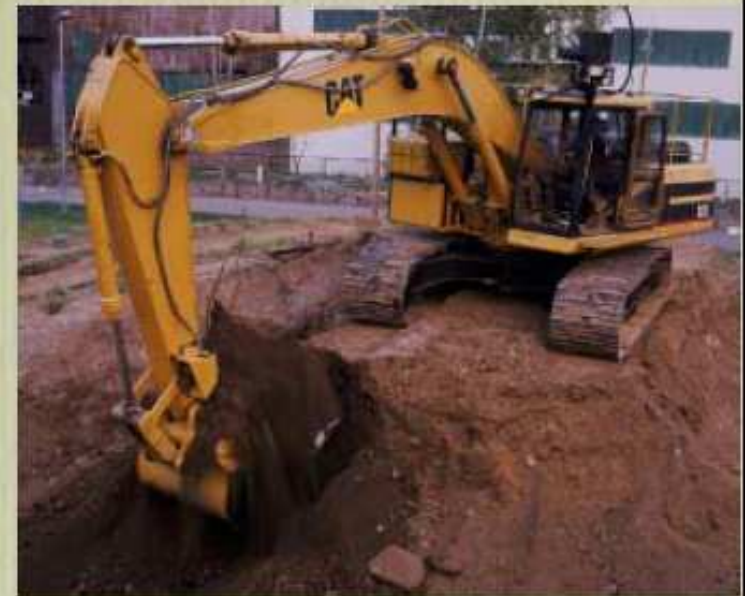
Fully Autonomous Excavator Truck Loading: Caterpillar/CMU
