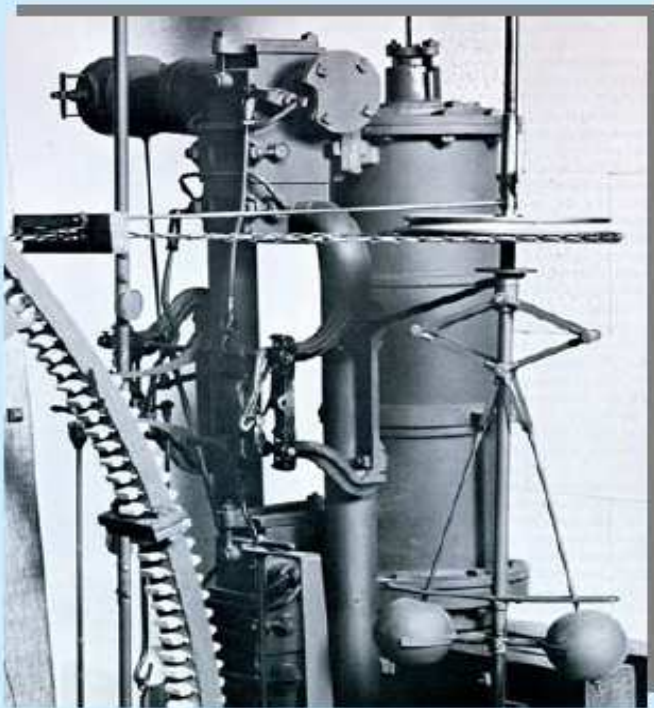
"Lap" (Steam) Engine, James Watt , 1788: continuous control operation
