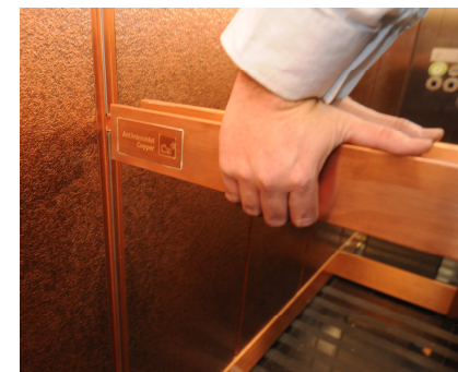
INSIDE LIFT HANDRAILS
